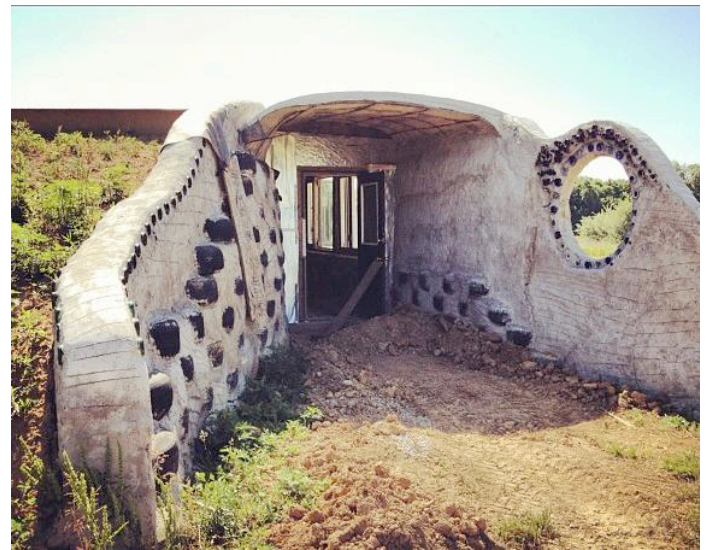
Sustainable Earthship made of old tires and mud
